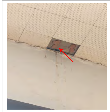
Closeup view of mastic pucks
